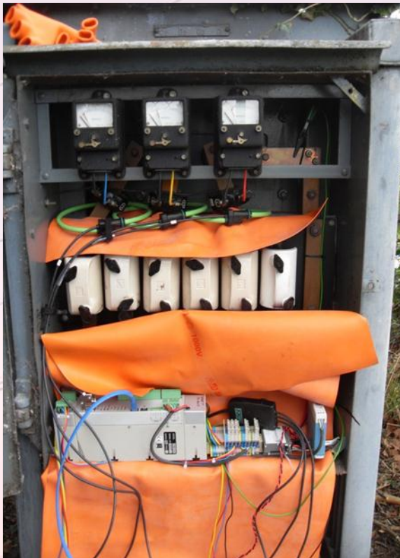
sub.net being installed
